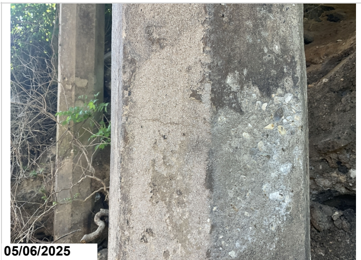
Bent 2 pile 2 cracks
