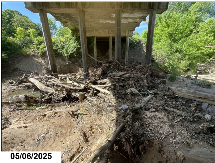
Span 2&3 drift
