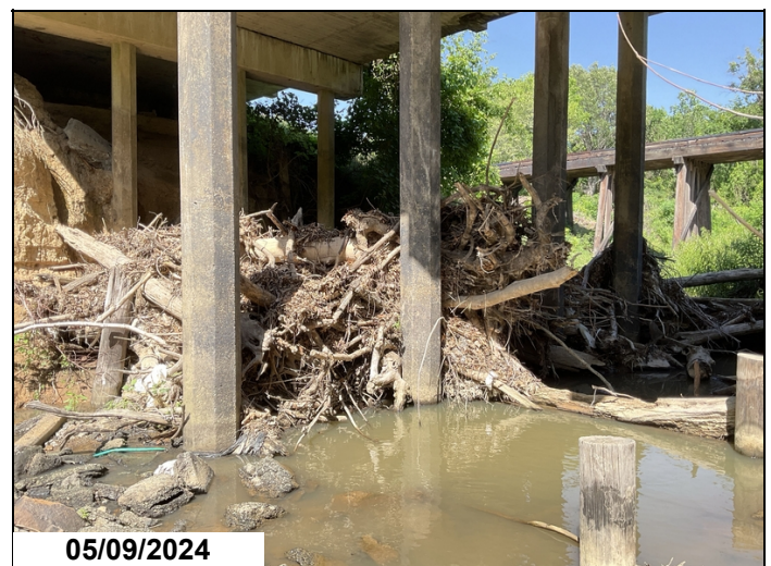
Bent 3 drift 19.5' of pile exposed from bottom of cap to ground line
