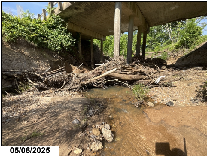
Span 2&3 drift
