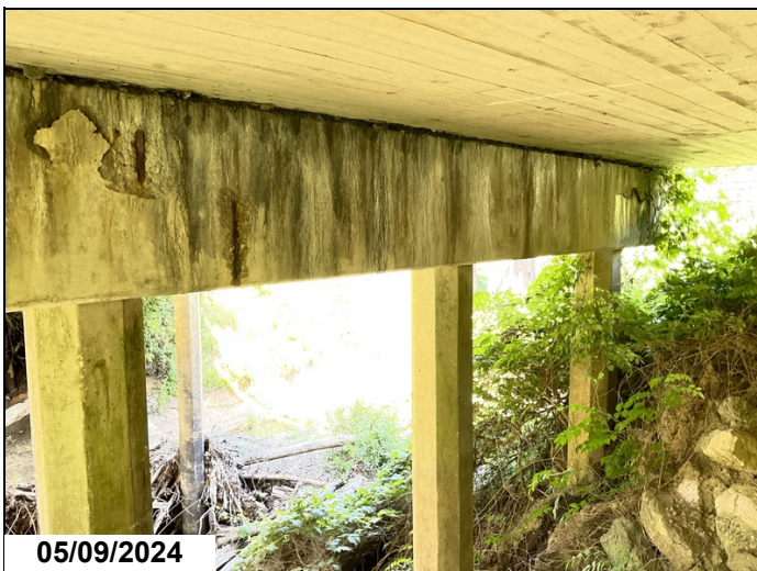
Bent 2 back side spalls and rebar CS3
