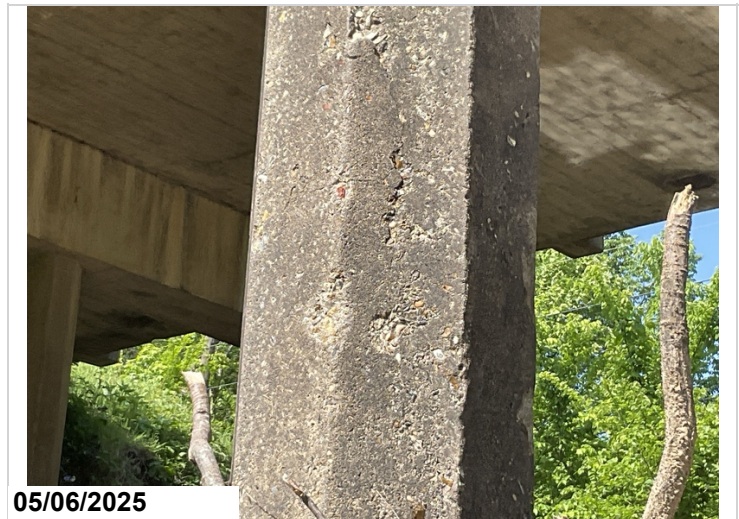
Bent 3 pile 4 horizontal and vertical cracks
