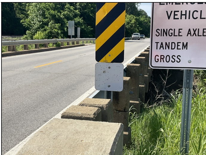
North end Log mile posting faded
