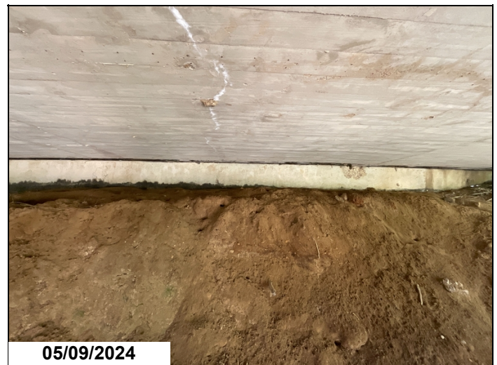
Bent 1 delam and minor chip/spall CS2 and 3
