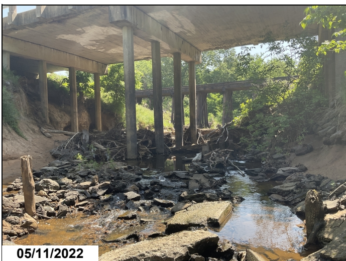
Span 2&3 drift
