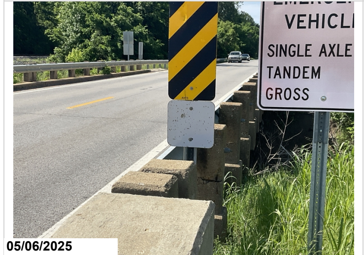
North end Log mile posting faded
