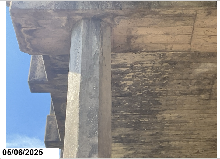
Bent 3 pile 4 vertical crack at top of pile
